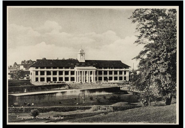
The Administration Block (Bowyer Block) of the General Hospital, early 20 th century.
